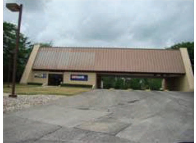
The US Bank parking lot has been patched many times and is in need of resurfacing.
