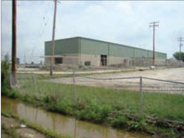
The fence around this industrial property is bent and falling down. Note drainage ditch running along side of the mall.
