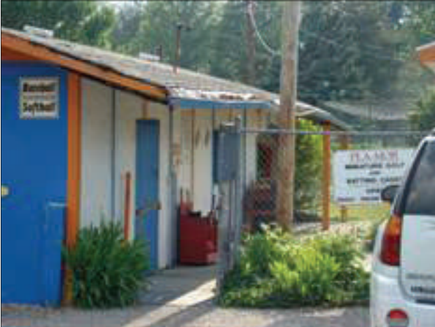
The roof structure on this building in the park is sagging in the rear corner.
