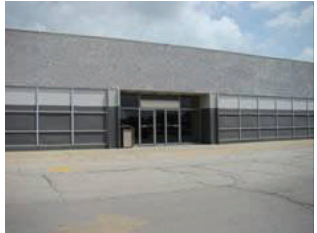
One of the larger vacant spaces at Cross County Mall.
