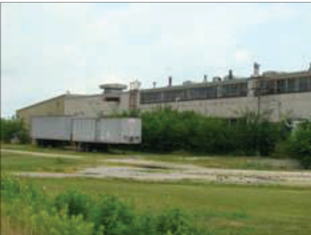
Semi-trailers are being stored on the overgrown rear loading area of the Alton lot. Note overgrown vegetation along the building's rear wall.
