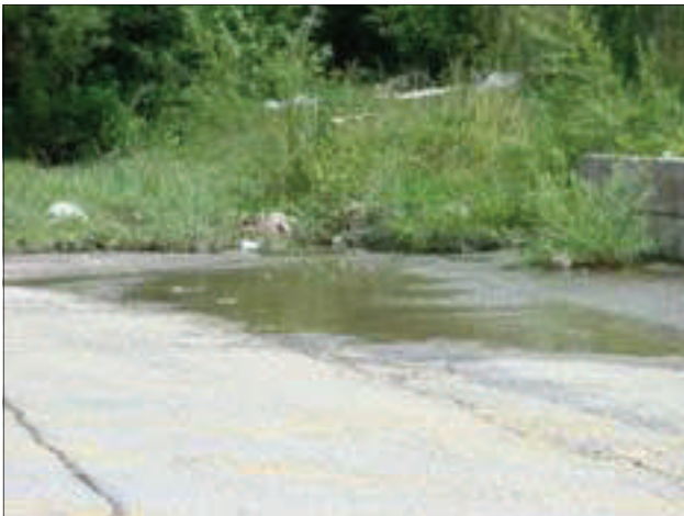
The storm drainage ditch in the rear of the mall overflows into the parking lot.
